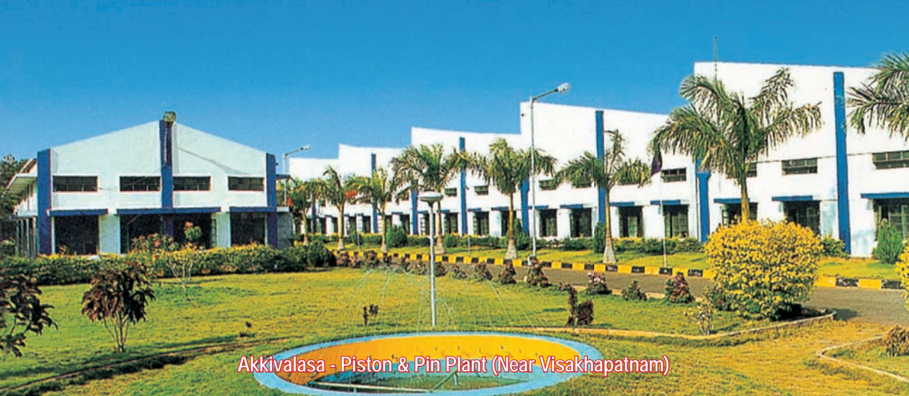
Varisam - Rings Plant (Near Visakhapatnam)
