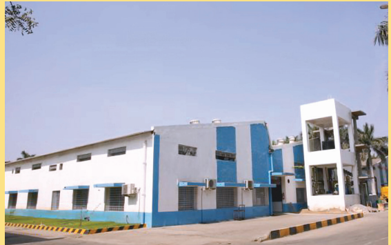
Plant 4, Bonthapally 79 Kms from Hyderabad Airport, Telangana
