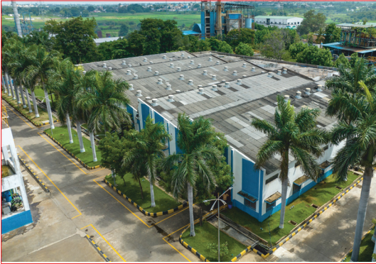
Plant 1, Bonthapally 79 Kms from Hyderabad Airport, Telangana
