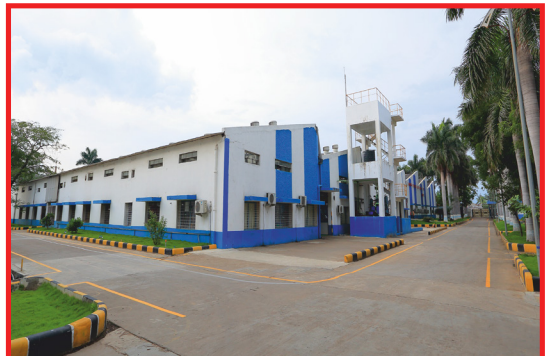
Plant 4, Bonthapally 79 Kms from Hyderabad Airport, Telangana
