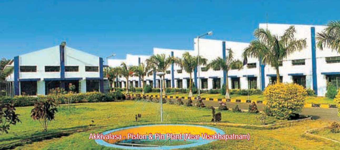
Varisam - Rings Plant (Near Visakhapatnam)
